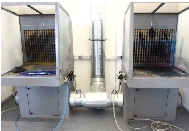
F.143 Spray finish booths with a strong exhaust system
