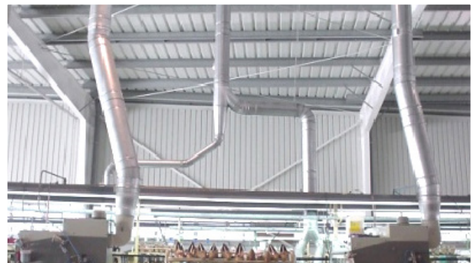
F.5 Exhaust system in a footwear factory
